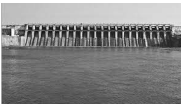
Plate 14 : Bargi Dam, Madhya
